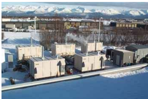
Figure 3.814 1MW power plant in Alaska (5 PEMFC 200 kW units in parallel)
