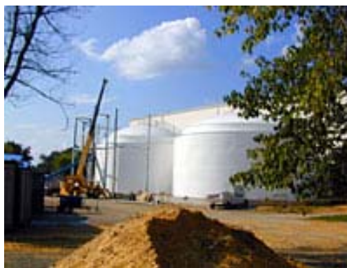
Figure 3.11 Electrolyte tanks of the TVA Regenesys plant under construction in Mississippi
