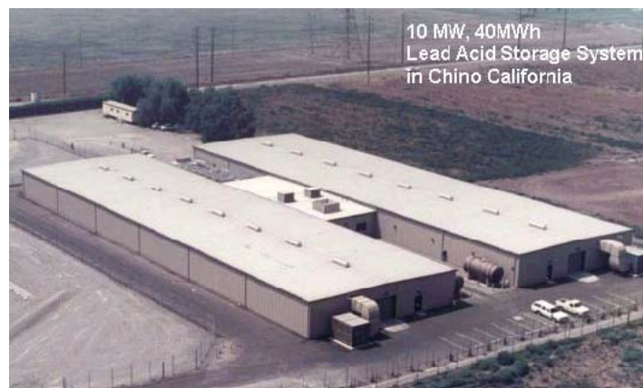
Figure 3.6 10MW/40MWh Lead-Acid storage system in Chino, California
