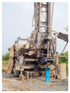
Figure 14: Water well being drilled
